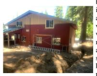
been rerouted, and fire sprinklers are currently being installed. New furnaces and duct work installations are in progress, and some of the rough electrical work is already in. Other changes include new windows for the new upstairs living spaces, masonry work to fill in openings no longer needed and a lot of deep holes and trenches for the new sprinkler systems and wire rerouting. We are still hoping to have the station livable again in another month or so.
